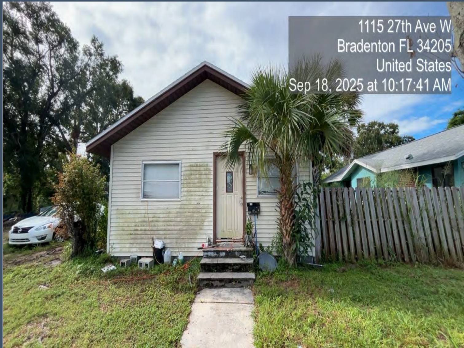
Street view of structure
